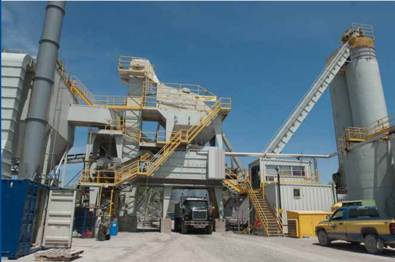
Walker Brothers Asphalt
