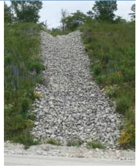
Rip Rap Drainage Ditch
