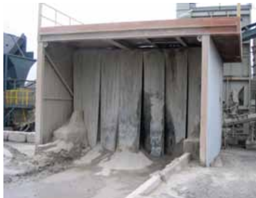
Agglime Storage Building
